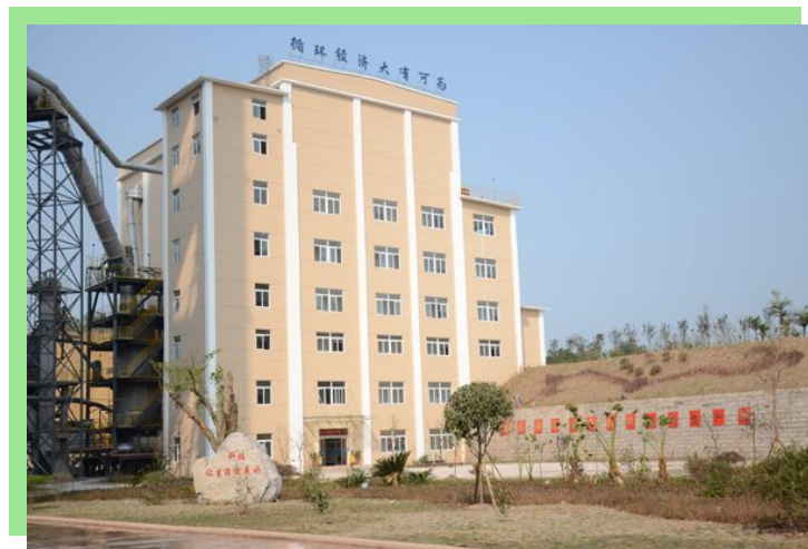
On April 11 2015, the waste incineration project in Zhong County of Chongqing completed construction and was put into operation.
