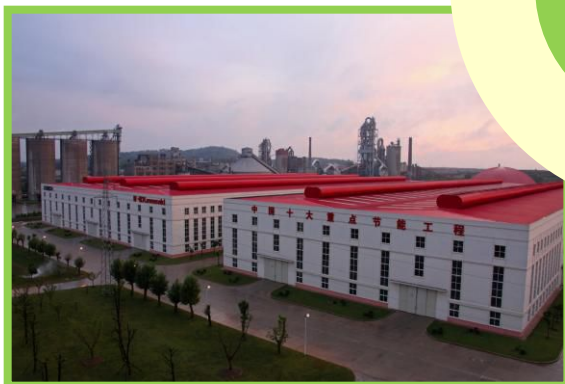
Residual heat power generation and Vertical mills
